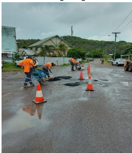
Pothole patching Douglas Street
