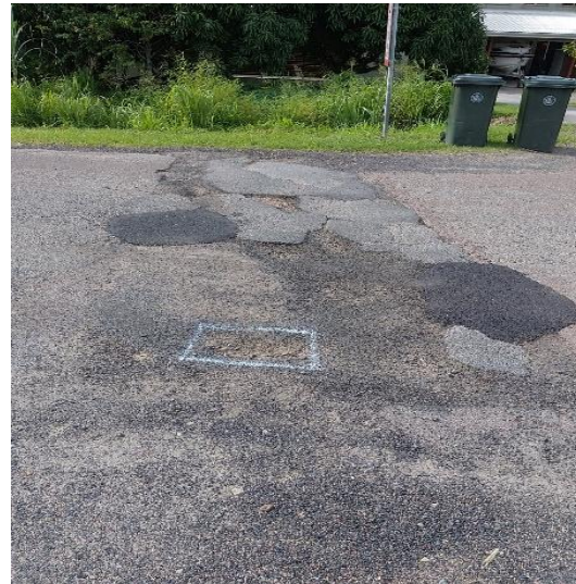
Pothole patching Hargrave Street
