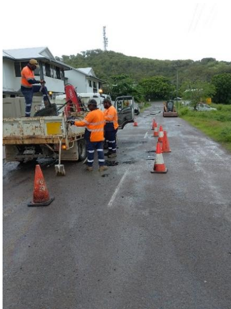
Pothole Patching Douglas Street
