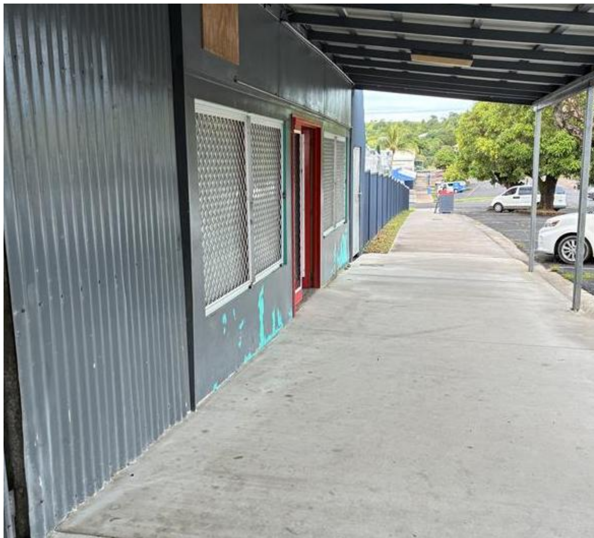
Figure 2 79 Douglas Street Building Frontage
